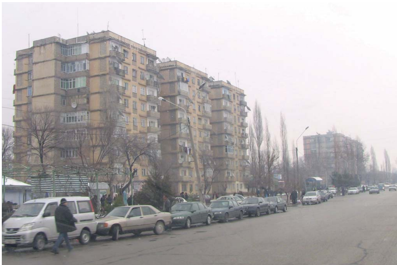
Picture 8. Multifamily housing in need of upgrading
