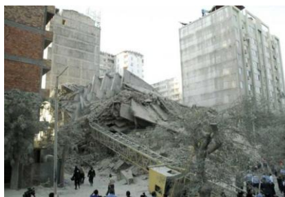
Picture 10. Demolished building after earthquake in Baku, August 2007 Source: Day.az
