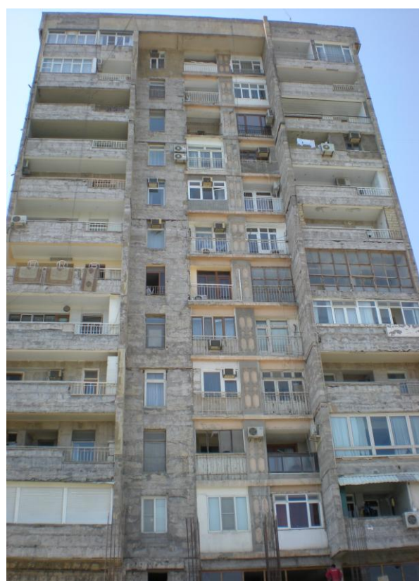
Picture 4. Façade of an apartment house in Baku
