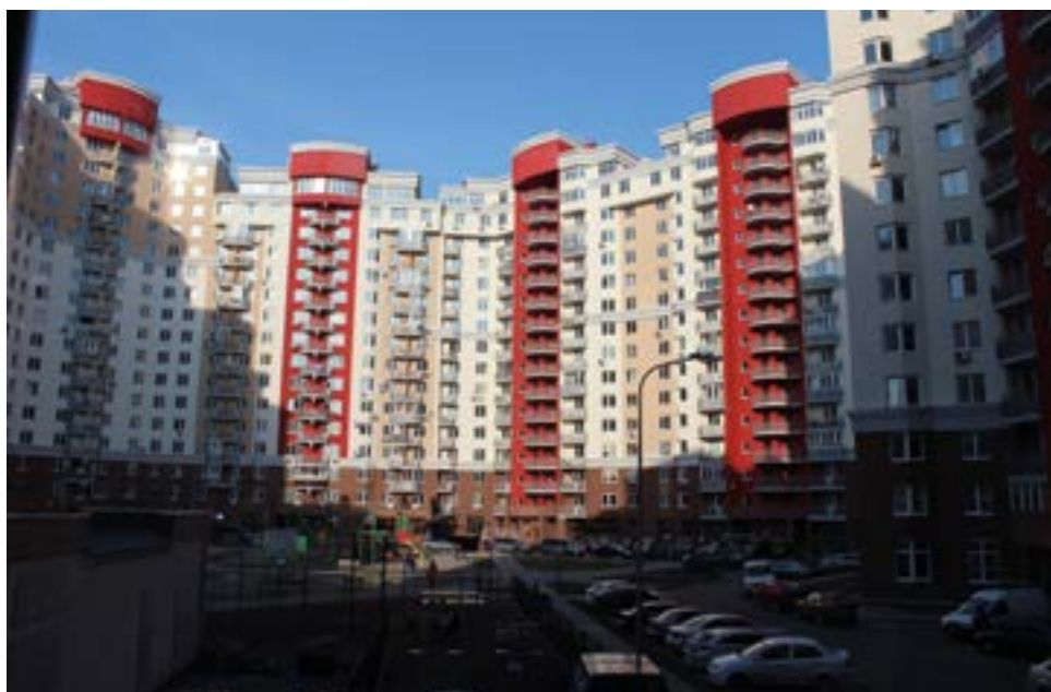
Picture 7. Rows of multi-apartment buildings with playground and parking
