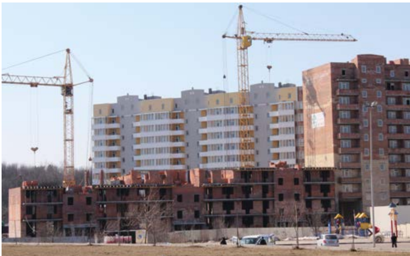
Picture 8. An apartment building under construction
