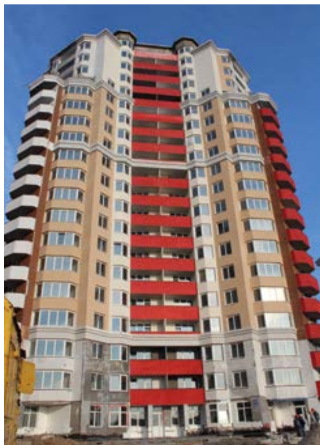
Picture 5. A social housing under construction
