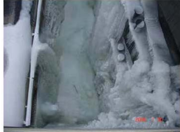
Ice occurrence in locks on the Danube preventing their operation. Source: via donau.
