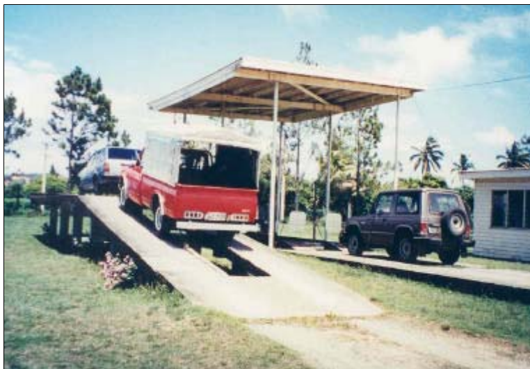
Plate 1: Simple low cost inspection ramp in Fiji.
