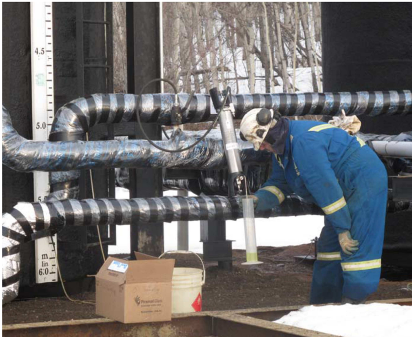
Figure 3: Pressurized Sample Collection at a Battery Site
